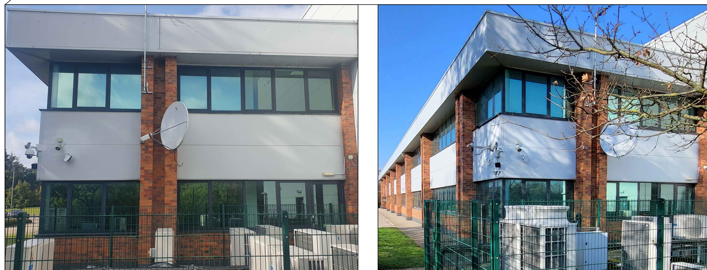
Example Images for new office elevation, following demolition of office structure, to line through and match west elevation.
